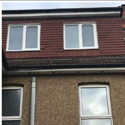
Missing wall hung tiles.
