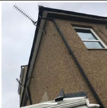
Fascia and soffit are not finished properly.
